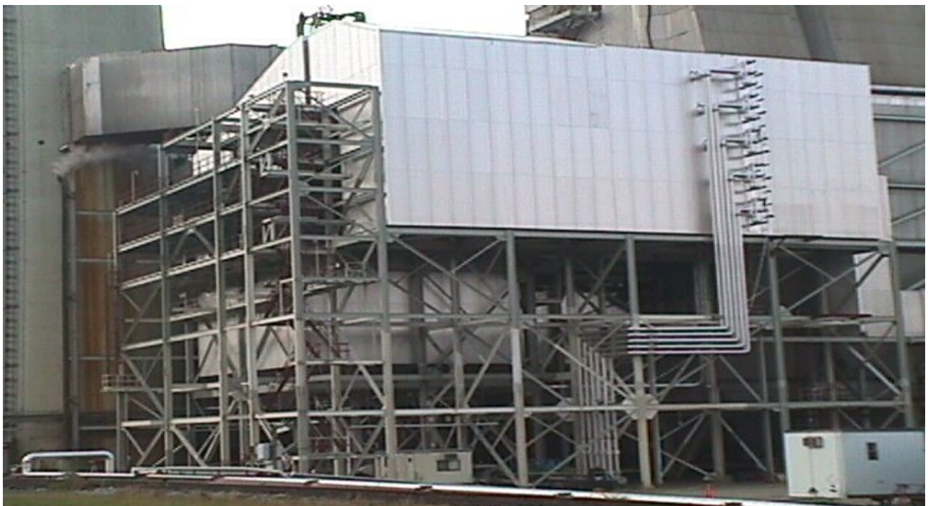
Figure 2: Flue at West Precipitator Exit – Note AIG
