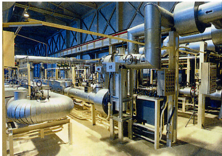
Figure.9 Bench Scale test facility and test condition
