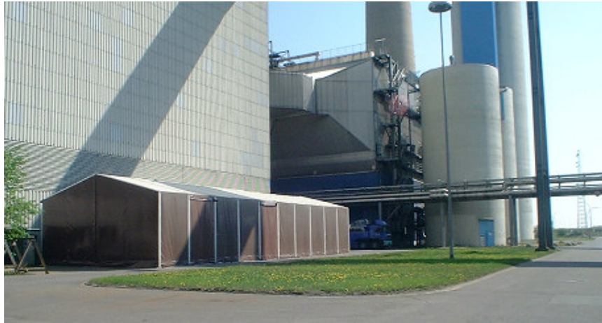
Figure 4: Working tent located by boiler house
