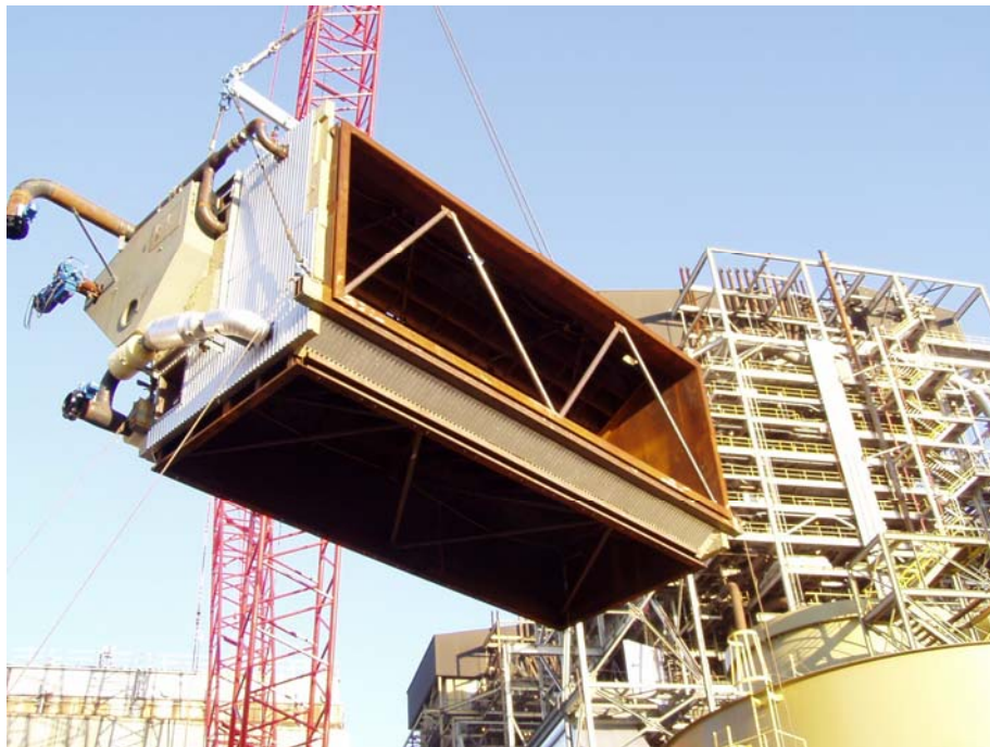
Figure 11 – Diverter Damper Being Lifted into Place (October 2007 Outage)
