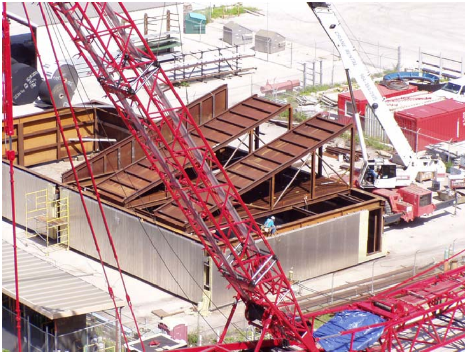
Figure 10 – Ground Fabrication of Reactor (top catalyst layer with inlet hood)
