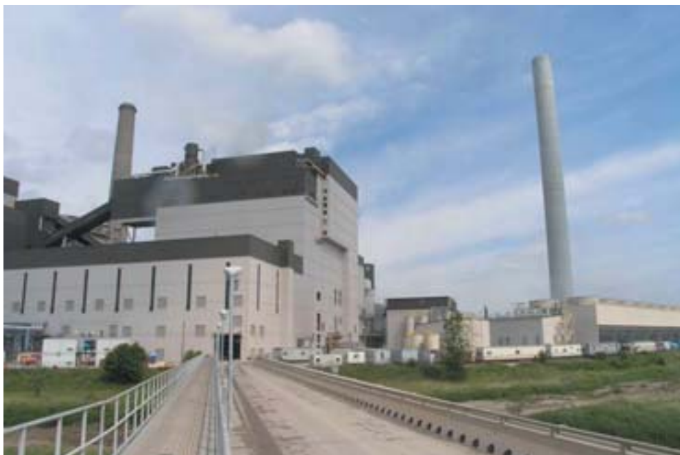
MidAmerican Energy: Walter Scott, Jr. Energy Center Unit 4 (USA) 850MW coal-fired once through boiler
