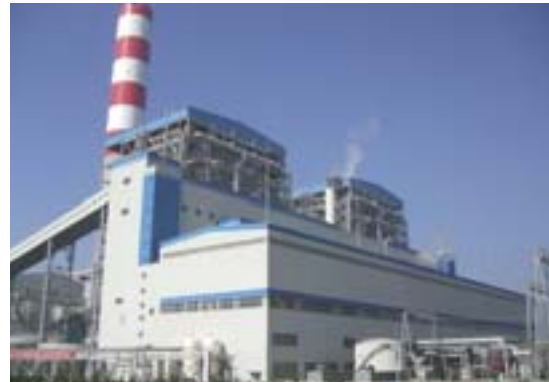
Wang-Qu No.1, 2 Shaxi Lulin Wang-Qu Power Co., Ltd. (China) 600MW coal-fired once through boiler
