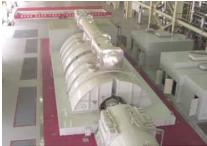
Turbine and generator for ShanXi Power Generation Co., Ltd (China) Wang-Qu Power Station No.1, 2 600MW, TC4F-40, 3,000 rpm 24.5 MPa, 566/566°C Generator capacity: 750MVA Put into service: 2006
