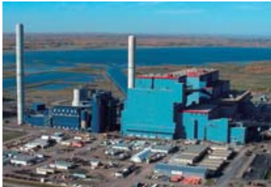
EPCOR Genesee Unit 3 (Canada) 450MW coal-fired once through boiler
