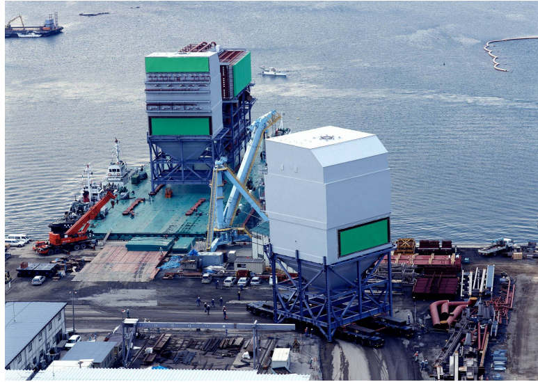
Figure-11 Transportation of GGH Modules
